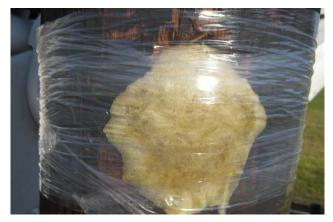
Woodpecker damage repaired with UPR™ Pole Repair
