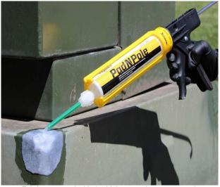
Fabric saturated with the high-strength, two-part resin creates a permanent Pad N Pole Repair.
