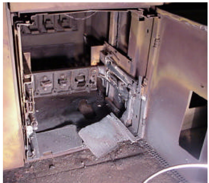
Figure 1: Arc Flash in a Floor Level Compartment
